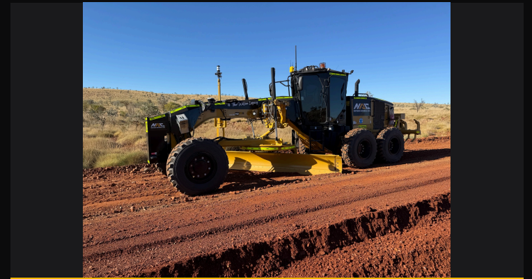
150 AWD Graders with Trimble Machine Control
